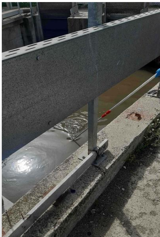
Sampling in WWTP Plovdiv
