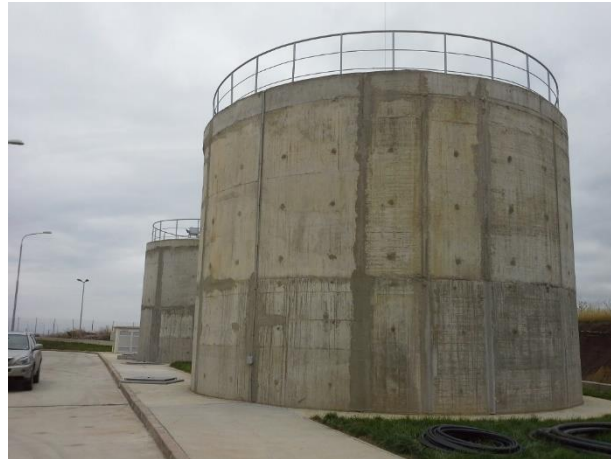
Fig. 2 Wastewater treatment plant "Sadinata"
