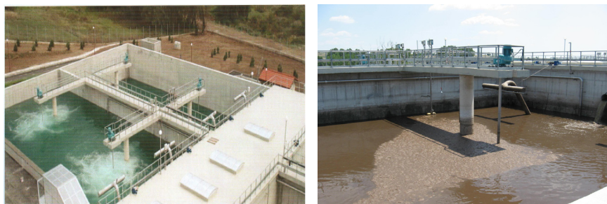
Figure 1. SBR aeration basins of WWTP-Hisarya.
